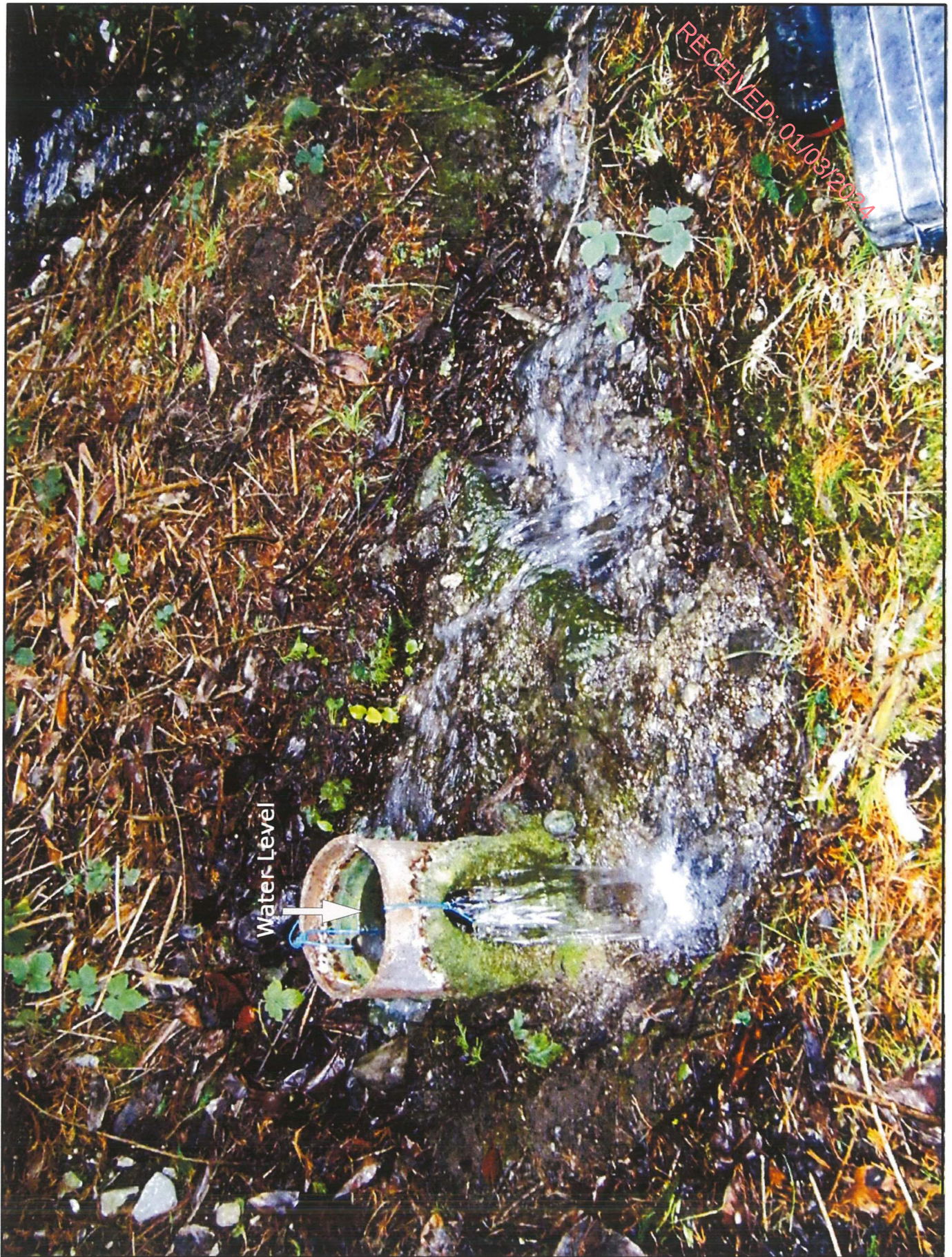
Figure 5.16 Flow from Borehole SG4 before a flange was installed on the wellhead.
